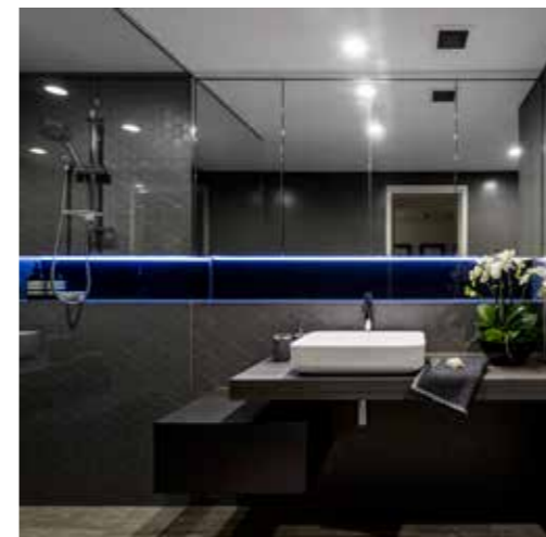
A built-out half wall concealing services and creating a utility shelf is continued into the shower in this bathroom makeover.
